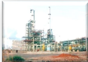
Gas Processing Unit at CBR & CBR Expansion 1 MMTPA
