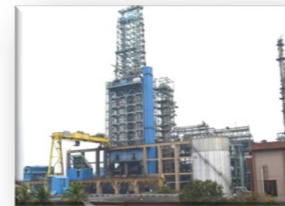
Resid Up-gradation [2.2 MMTPA DCU]
