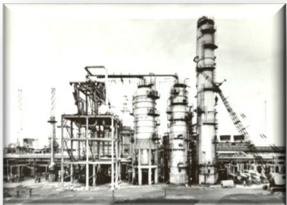
Ref-I – 2.5 MMTPA + Lube Oil Block Commissioned
