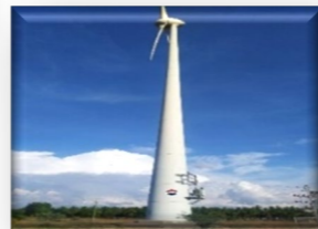
Wind Mill 17.6 MW
